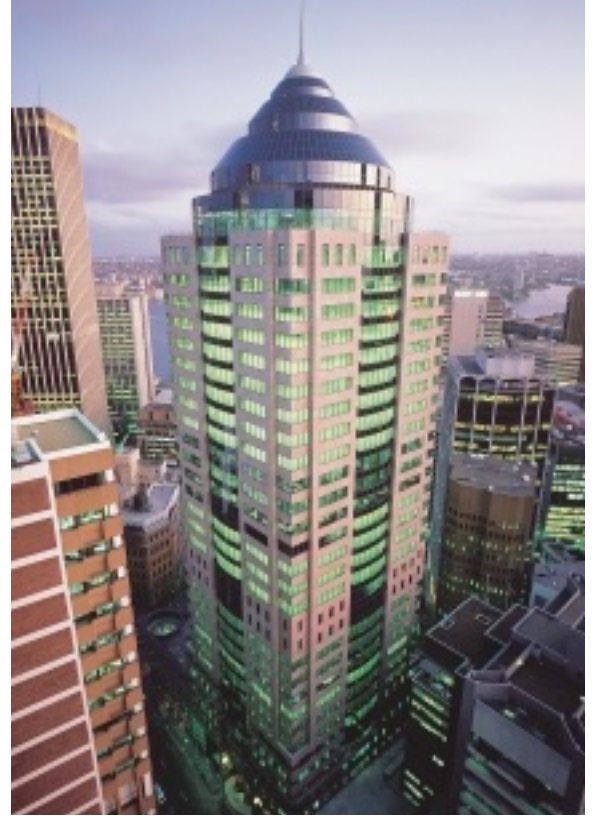
CITY SPACE The AGSM takes up residence at 1 O'Connell Street, Sydney.
